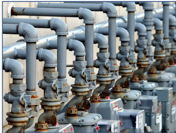
Residential gas meters on the side of an apartment building Photo Credit: Flickr Creative Commons / mkrigsmann
